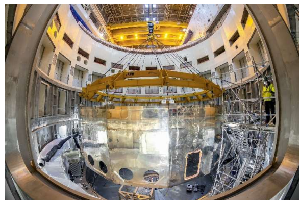
Installation ongoing in the ITER Tokamak Pit
