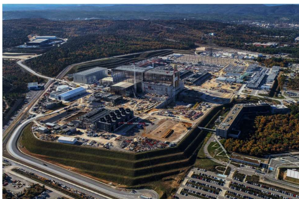
Overview of the ITER worksite
